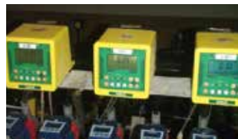
⑤ Nourishment control equipment
